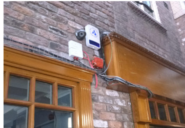
Poorly sited exposed wires and equipment.
