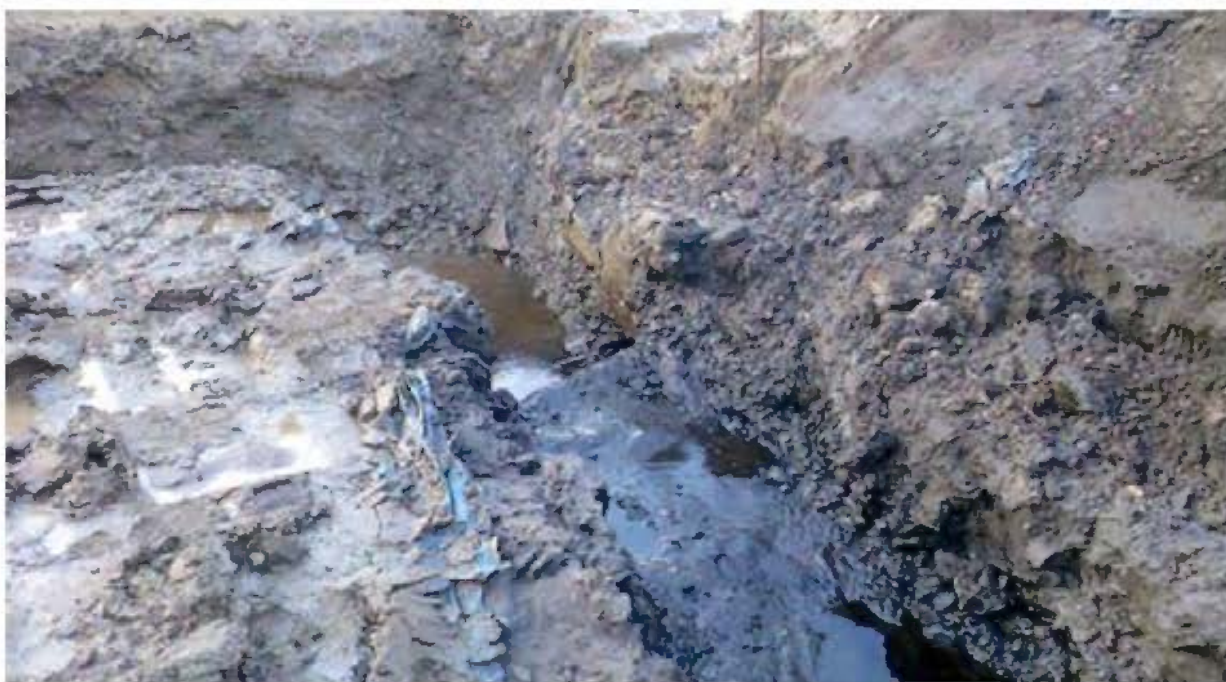
Photograph 4: Hydrocarbon impacted soils and water within foundation excavation.
