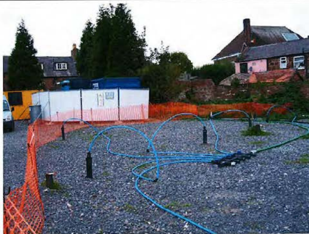
Plate No.: 54 Title: Multi-Phase Extraction Treatment System Connected to Treatment Wells
