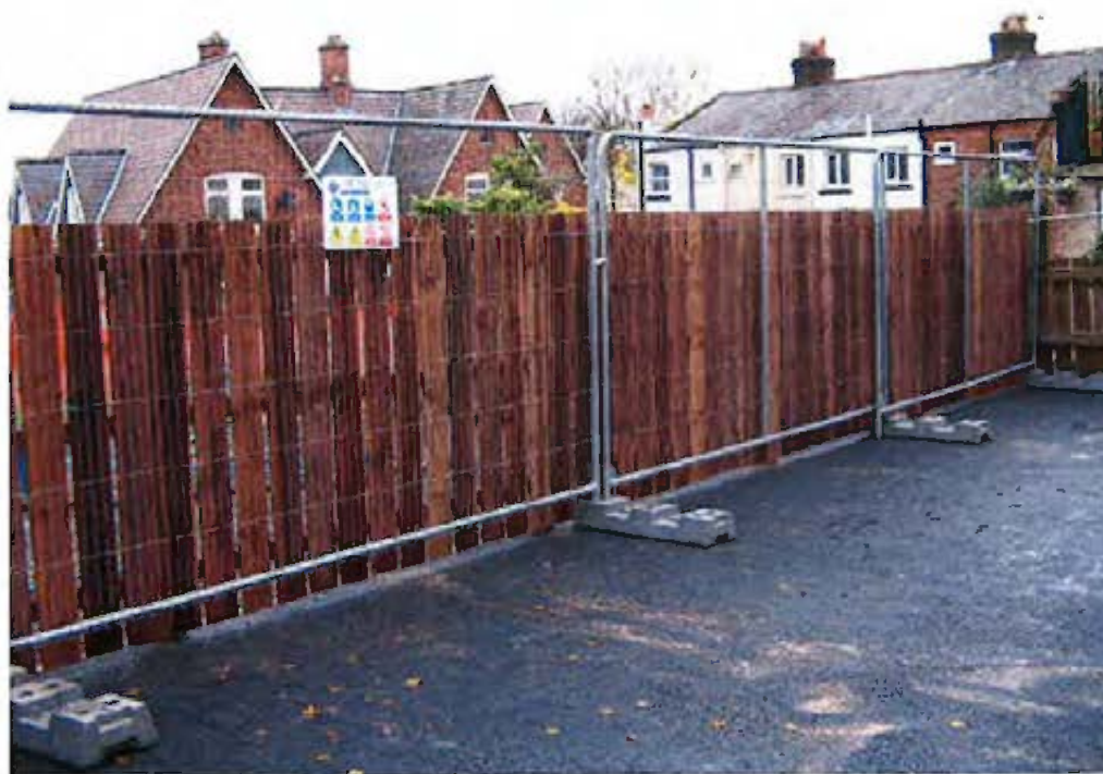
Plate No.: 58 Title: Reinstated Wooden Fence with Mesh Fencing to Prevent Trespasses to Site
