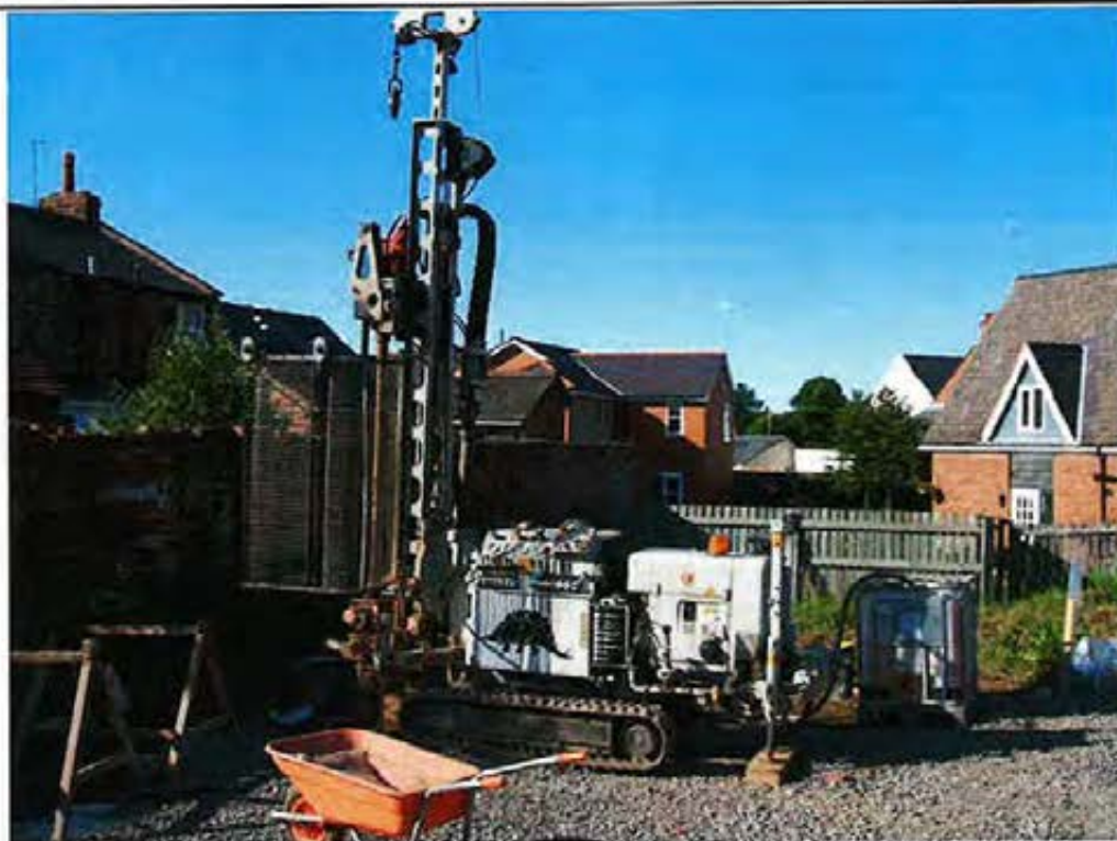
Plate No.: 41 Title: Rotary rig setup at borehole location CTW3
