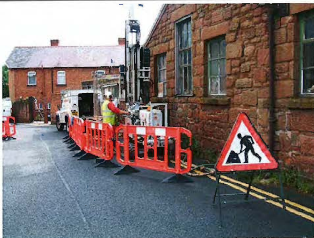
Plate No.: 42 Title: Rotary rig setup at borehole location CB12
