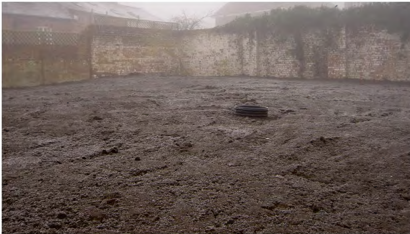
Photograph 4: Hydrocarbon impacted soils and water within foundation excavation.
