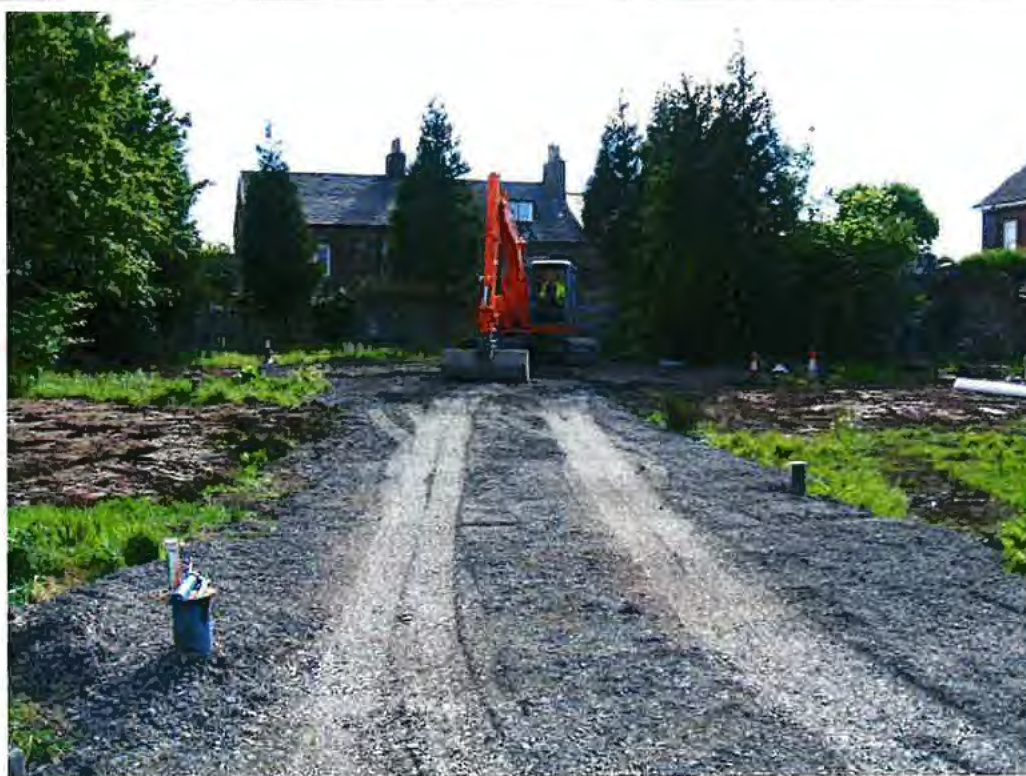
Plate No.: 38 Title: Access road to treatment pad with 200 mm thick of clean lime stone
