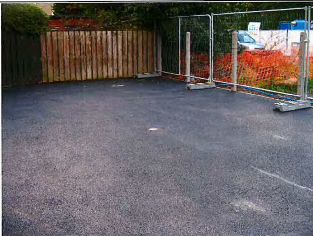
Plate No.: 57 Title: No. 5 and 5A Cross Street Back Garden After Tarmac Reinstatement Works (Facing West)
