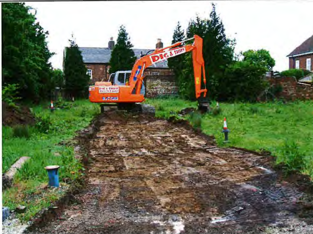
Plate No.: 37 Title: Removed top 200 mm of topsoil for access road to treatment pad.
