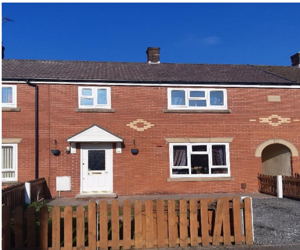
Typical roof refurbishment
