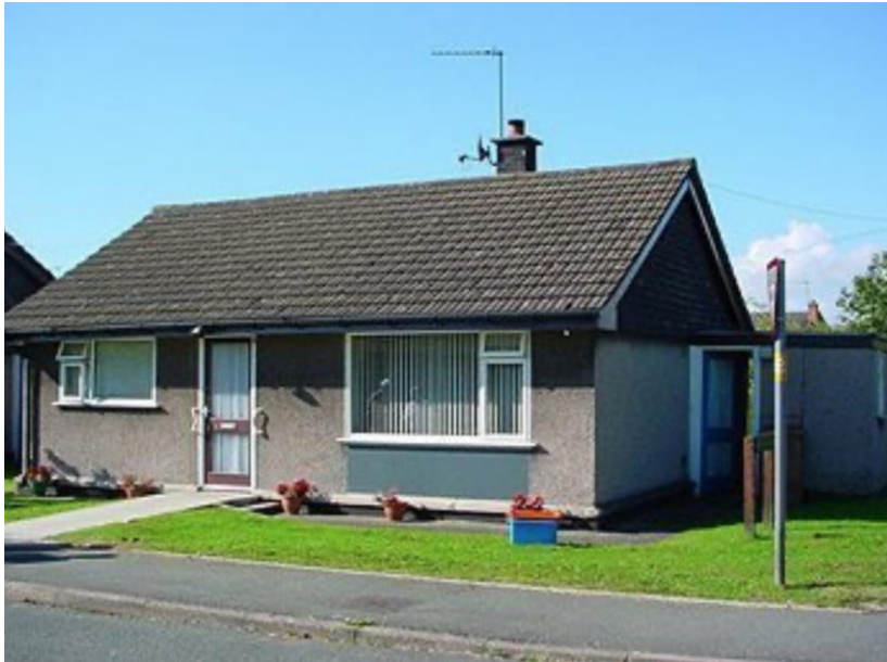
Typical Kencast Precast Concrete House
