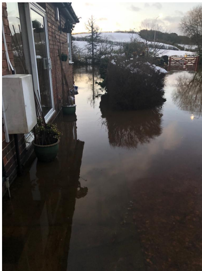
Figure 3 – Flooded Property on the A54
