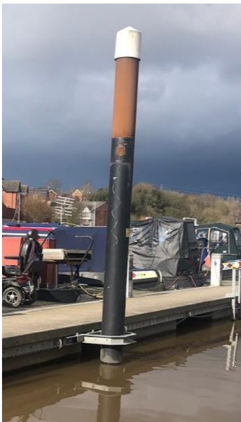
Figure 12 - Northwich Quay Pile. February 2020
