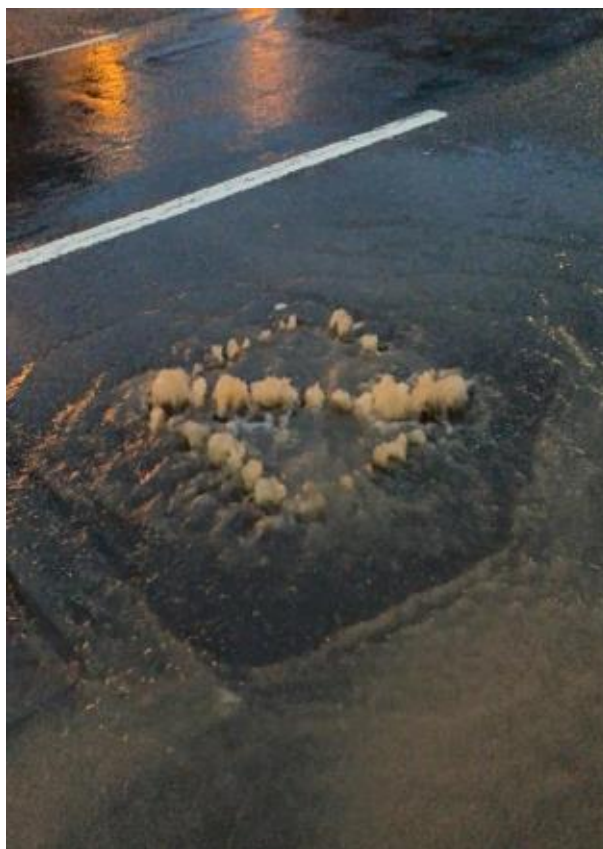
Figure 2 - High Street manhole cover opposite Old Mill Place. 20/01/21
