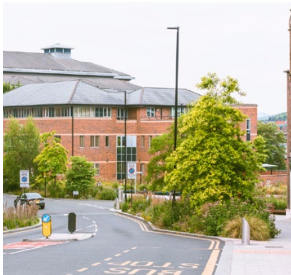
Example of how the underpass could have trees and planting to create an attractive environment at the junction of Northwich memorial Court. Image of Grey to Green, Sheffield
