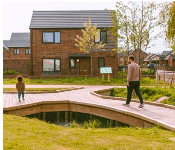
West Gorton Sponge Park - An example of a neighbourhood park with floodable areas and SuDS
