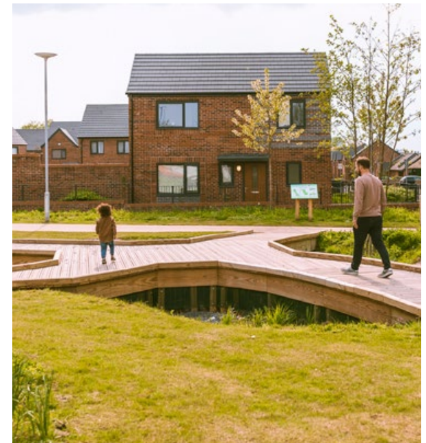
West Gorton Sponge Park - An example of a neighbourhood park with floodable areas and SuDS
