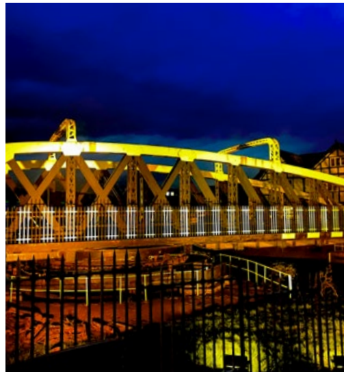
Grade II Town Bridge, Spanning the River Weaver and built by the Weaver Navigation Trustees in 1898-99
