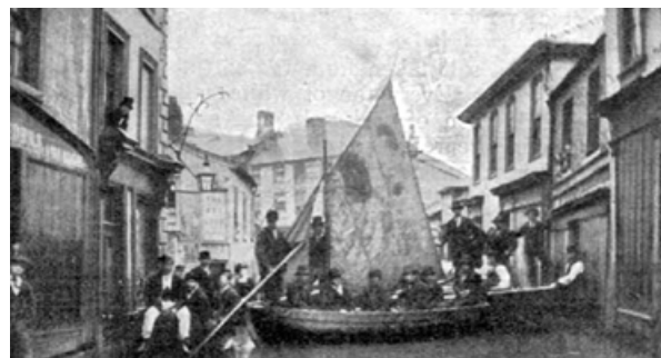
Flooding in Northwich
