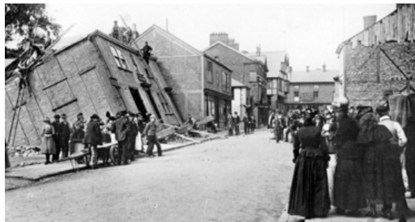
Subsidence in Castle Street, 1890 - 1899
