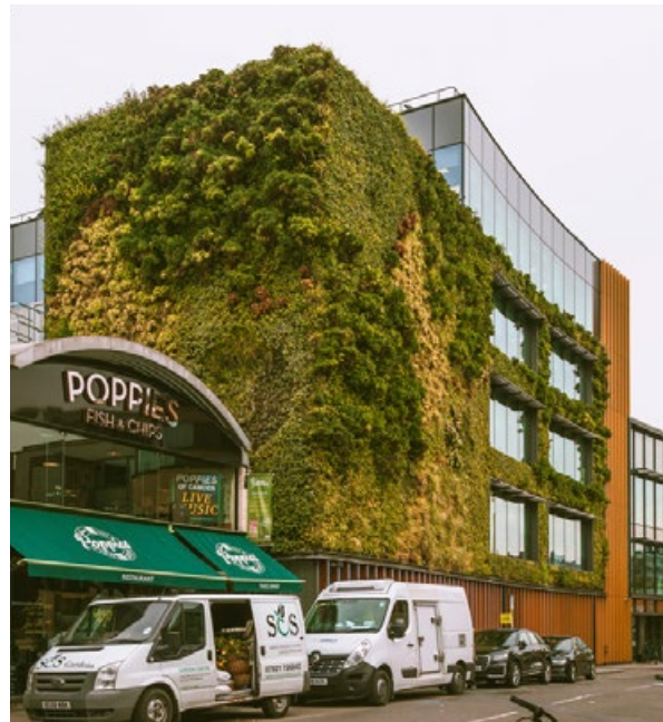
Green wall creates an attractive facade and improves the street environment
