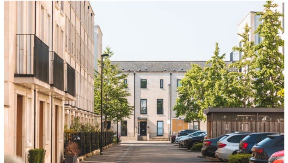
Car parking is overlooked by development, tree planting is integrated between parking to avoid cars dominating the street
