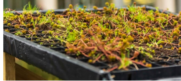
Green roofs with sedum planting to mitigate surface flooding
