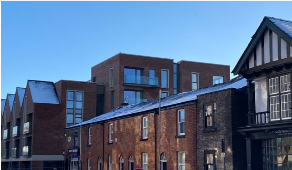
Sensitive design of new development next to heritage buildings
