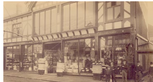
Timber framed buildings on Witton Street
