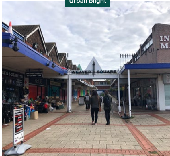
Weaver Square indoor market, dilapidated building, vacant retail units
