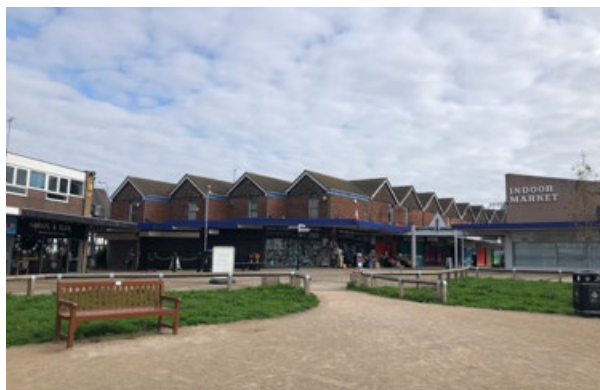
Weaver Square, green space where the outdoor market used to stand
