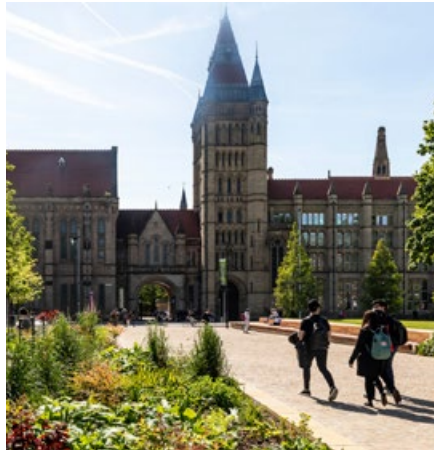
Example of a cultural building and a pedestrian crossing points
