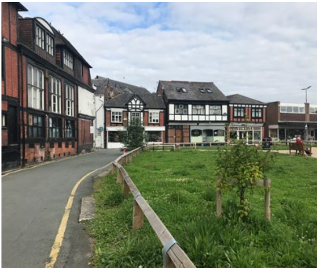
Locally listed buildings fronting Market Street
