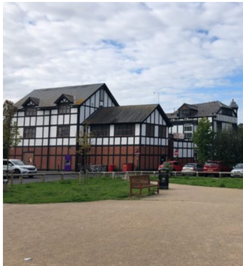
Rear of NatWest building from Apple Market Place
