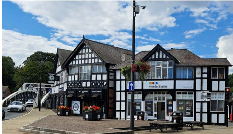
Grade II listed, Town Bridge and locally listed buildings contribute to the historic character of the Bull Ring, Northwich
