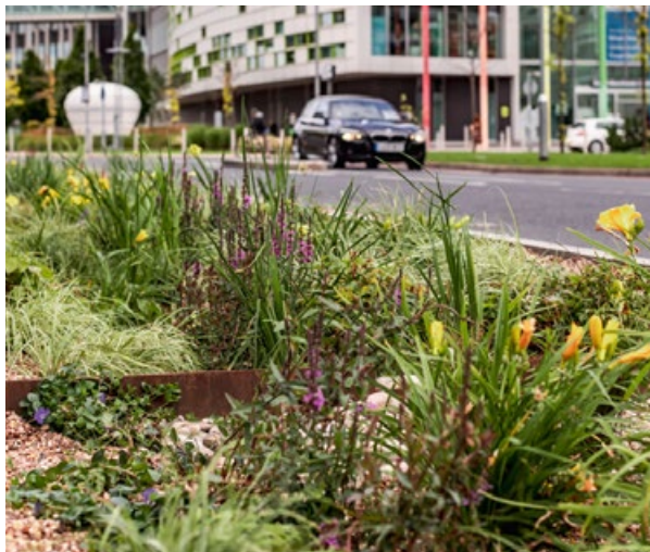
Raingardens adjacent to road to capture run-off
