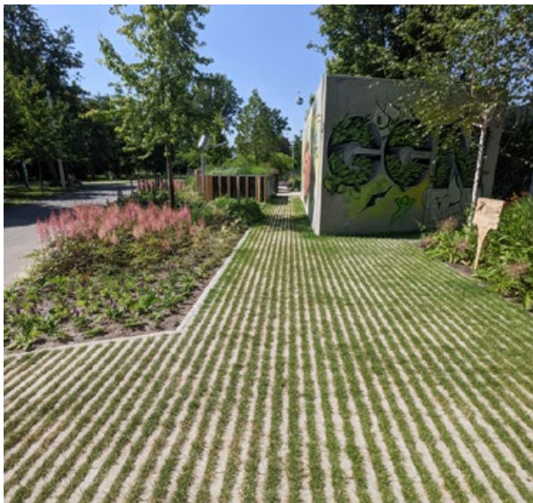
Grasscrete - incorporating turf into parking areas and / or shared spaces to alleviate flooding
