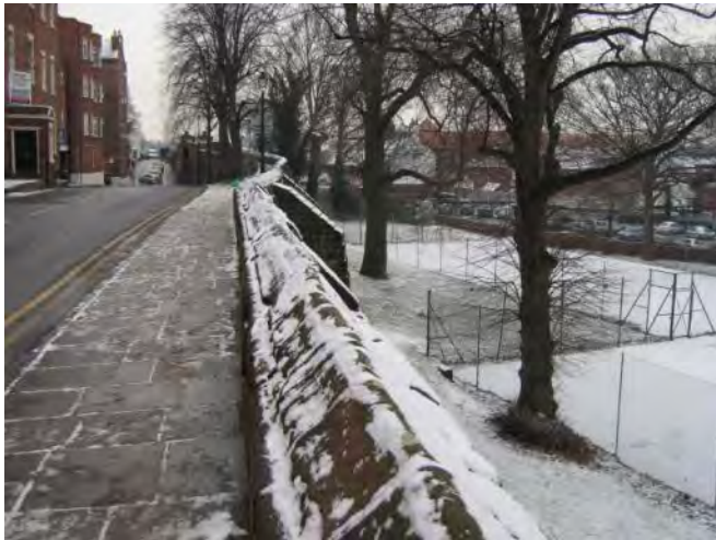
The dramatic change in level across the western wall
