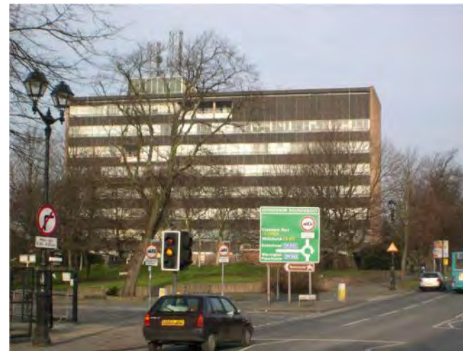
Former Police HQ Building
