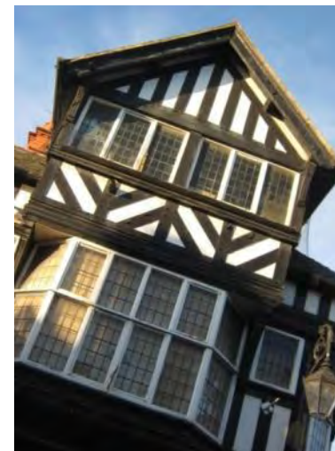
F2b. 53 Frodsham Street – a 3 storey Vernacular Revival style property with oriel window
