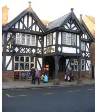
F1f. 97 Foregate Street 9 (The Old Queen's Head) - a two storey restored building in vernacular style, with projecting central bay on timber piers
