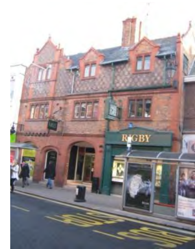
F2a. 12-14 Frodsham Street – a 3 storey, Victorian red brick building with decorative brickwork at upper level, arches at ground floor, and recessed mullion windows
