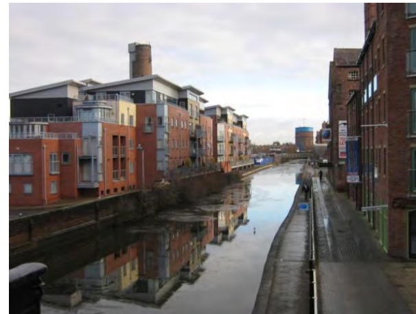
City Road Bridge to Hoole Lane (G3)
