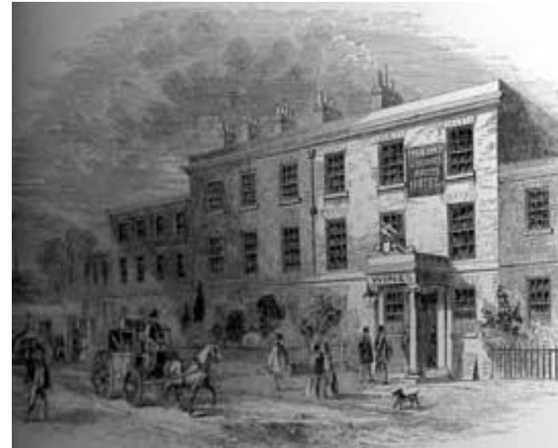
Liverpool Arms Hotel (now Lloyds Hotel), Brook Street, 1856
