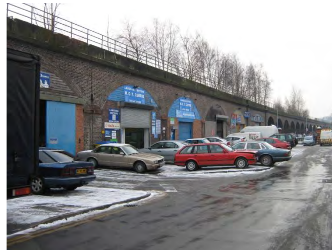
The Railway Viaduct Arches
