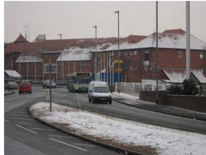
Poor frontage along New Crane Street
