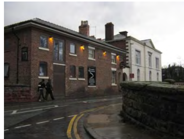
Telford's Public House and the former canal company offices
