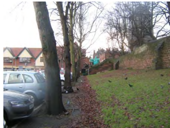
Kaleyards car park and the City Walls
