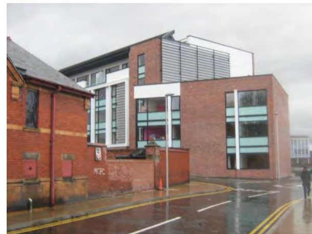
Modern residential development
