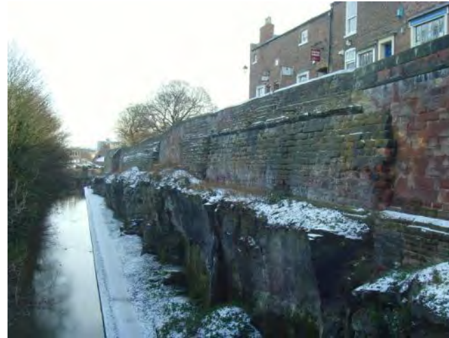
City Walls at Northgate Canal Cutting
