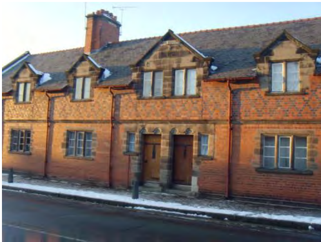
Gothic Revival terrace on Overleigh Road
