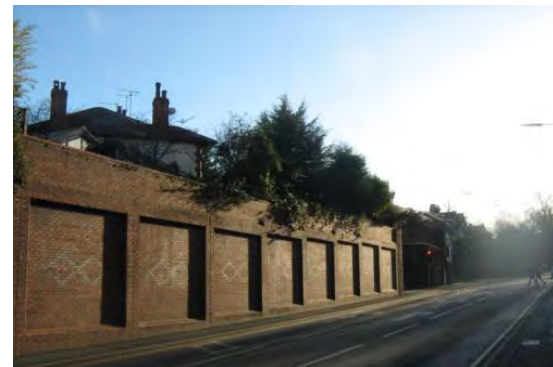
Retaining walls along Parkgate Road
