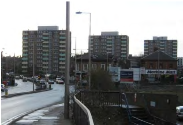
The three tower blocks of St Anne's, St Oswald's & St George's
