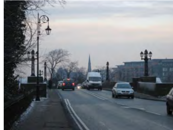
View of Grosvenor Bridge looking north towards the City
