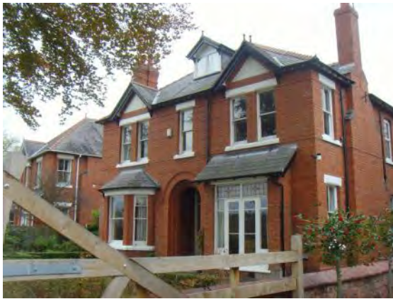
Typical Edwardian house in the area
