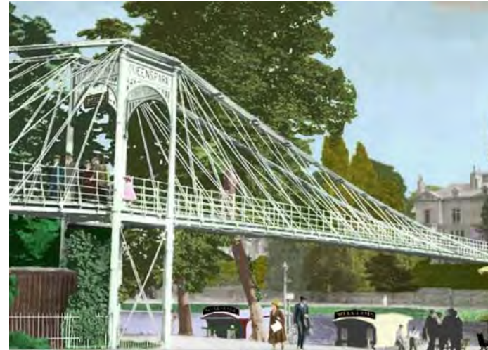
Original Queens Park Bridge 1920s (restoration by Jeremy Stubbs)
