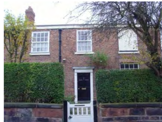
36 Chapel Street - a typical Georgian house
