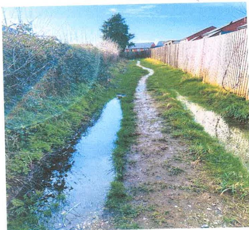
IMAGE 14: TRACK – Viewed from behind Substation (ESS) on Shearwater road looking towards Churton Road and erected fence. Photograph shows recent access on foot evident February 2020
