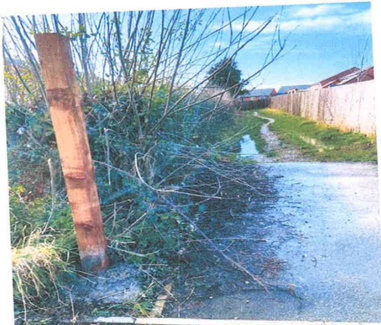
IMAGE 15: TRACK – Viewed from behind Substation (ESS) on Shearwater road looking towards Churton Road. Photograph shows new erected fence and recent access on foot evident February 2020
