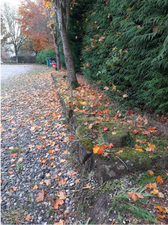
Diversion line of FP21 relocation of 2 trees, groundworks levelling
