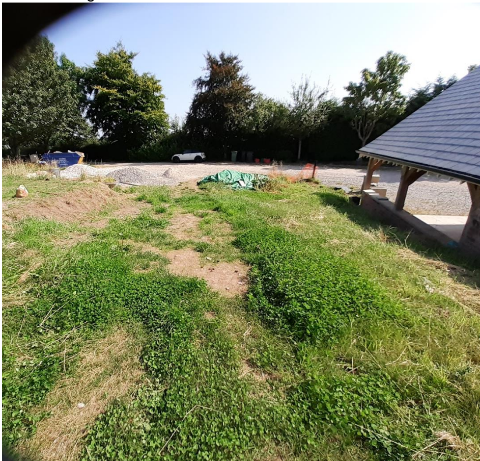
Proposed route of FP20 diversion avoiding guy cable. Levelling and gravel surfacing for FP20 diversion to connect with FP21 at line of trees in image.
