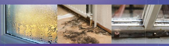
This leaflet explains how condensation forms and how you can keep it to a minimum and reduce the risk of dampness and mould growth.
