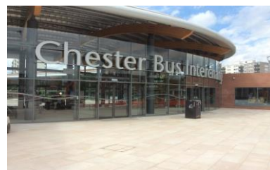
Chester Bus Interchange Entrance
