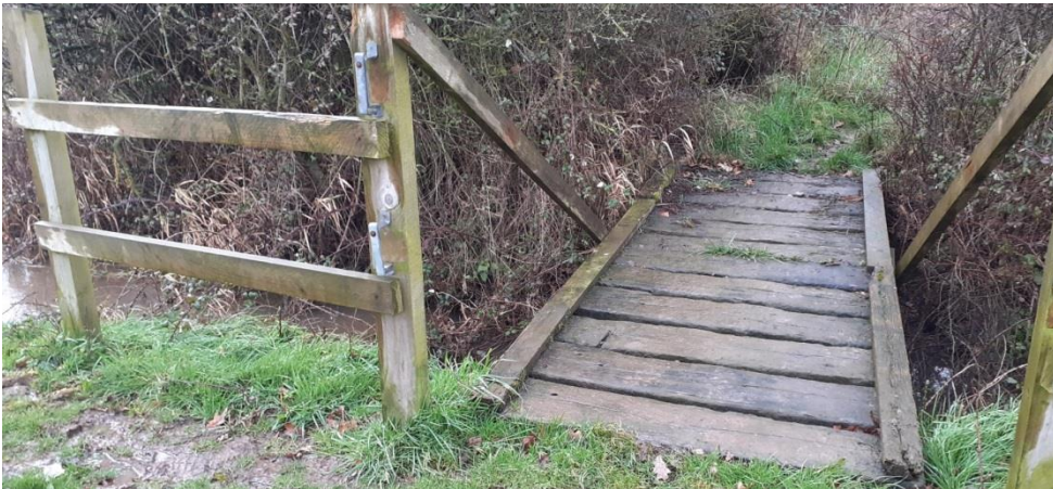
Diversion along side brook and foot bridge crossing at Point e
