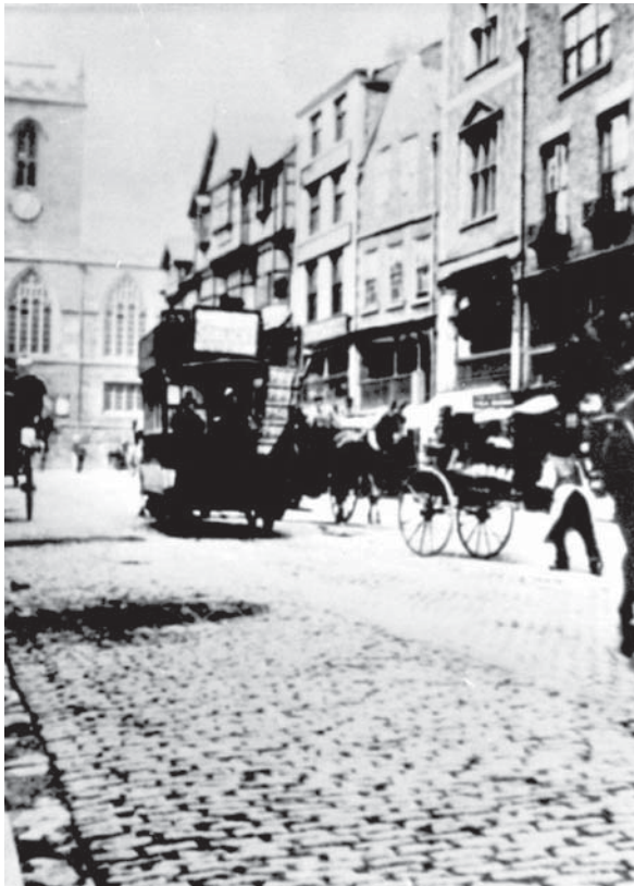
Setted carriageway to Bridge Street 1900
