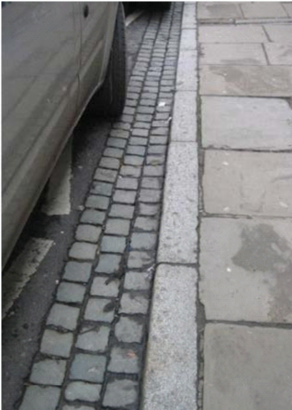
Example of granite kerb with setted channel detail
