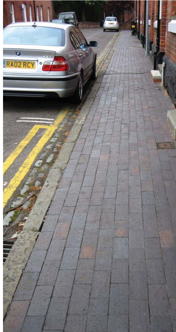
Blue clay pavers to footways in Albion Place
