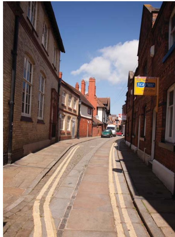
Traditional paving on Bunce Street
