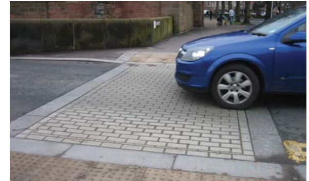
Example of type C1 – Courtesy crossing (using mastic asphalt imprint) at Bridgegate, Chester
