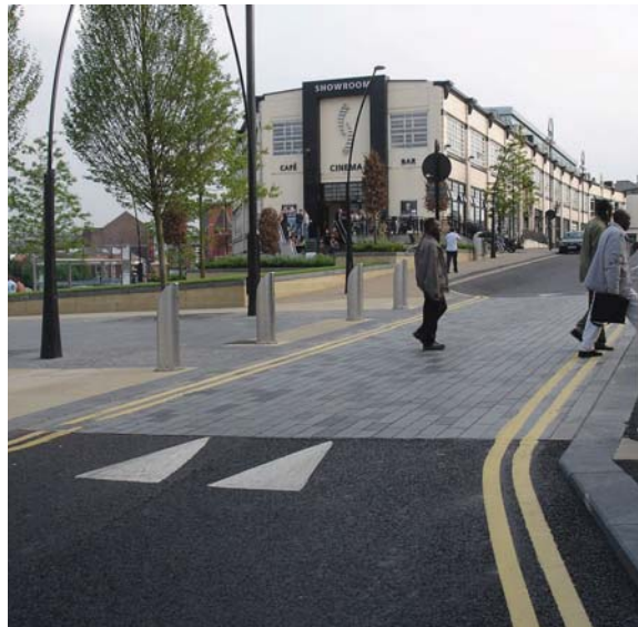
Good example of controlled crossing in granite setts, raised to kerb height
