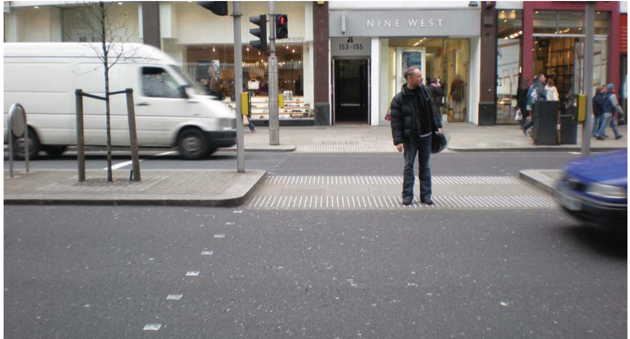
Good example of flush controlled crossing with no pedestrian guard rails
