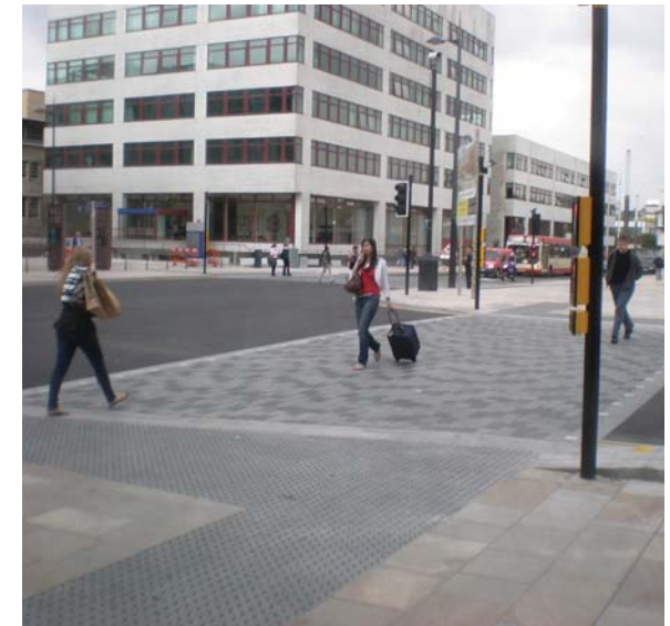
Good example of controlled crossing with granite setts on busy traffic route
