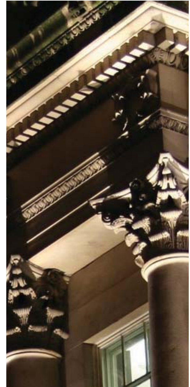
Lighting can be used to highlight architectural details that would otherwise be missed by many of us, and to add drama to our public spaces.
