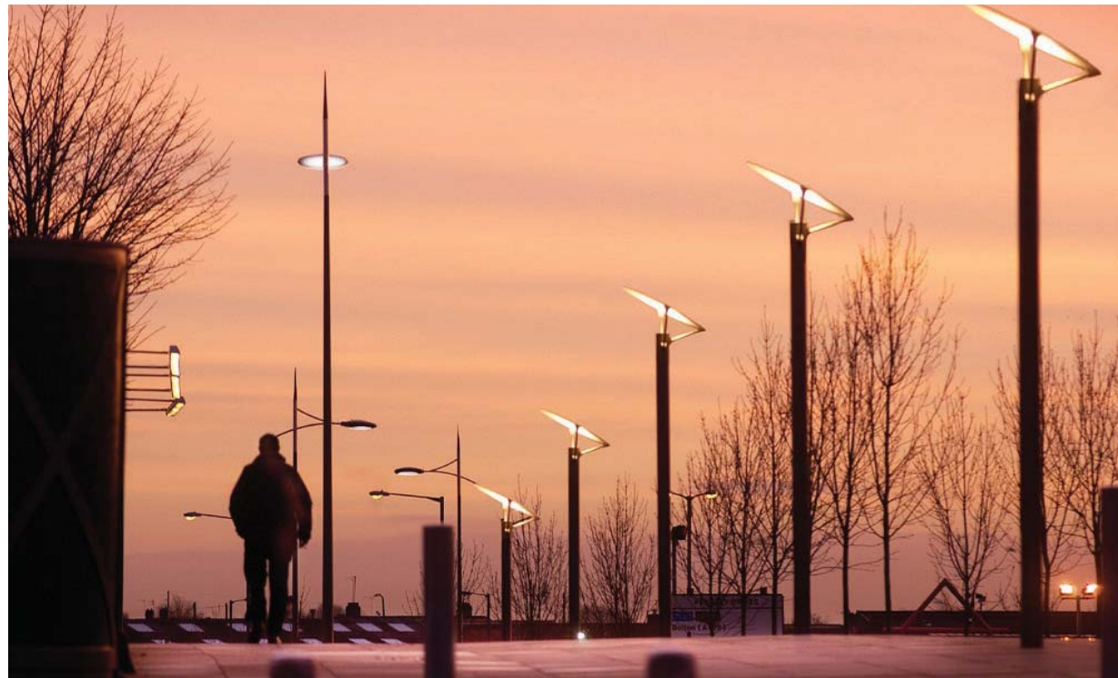
Street lighting positions, George Street, St Helens
