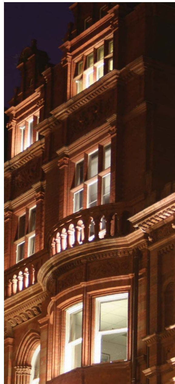
Good example of architectural lighting
