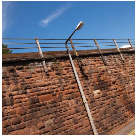
Older style / functional road lighting lanterns within the city walls – both lanterns and columns would benefit from renewal
