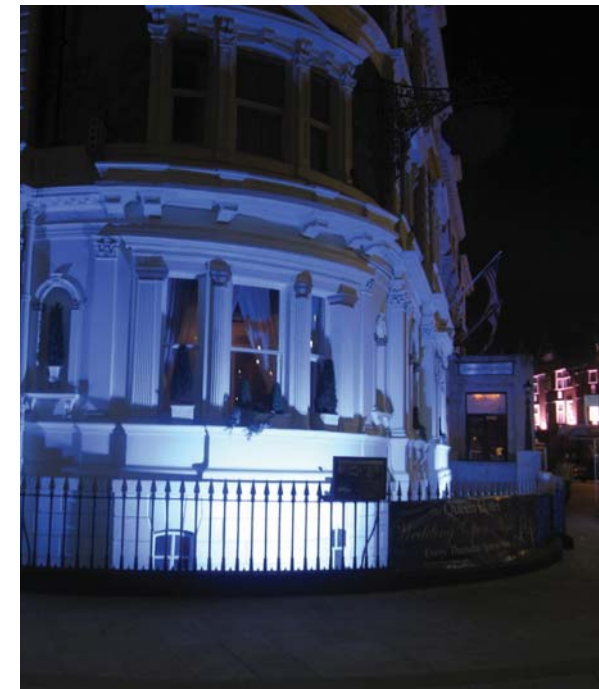
Poorly executed or inappropriate lighting has a negative impact. This hotel is the first thing seen when leaving the railway station and does little to promote the city in a dignified way.
