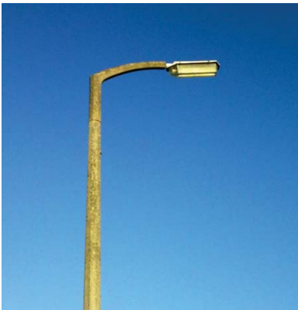
A typical flood light - although fairly discreet it could be less visible and the absence of any glare control is unacceptable
