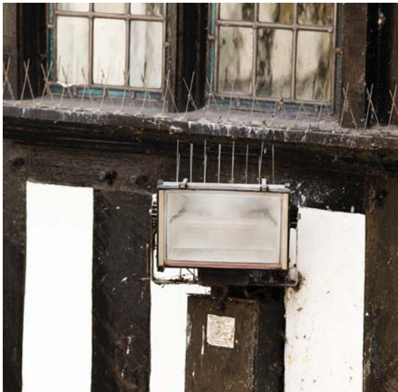
A typical flood light - although fairly discreet it could be less visible and the absence of any glare control is unacceptable
