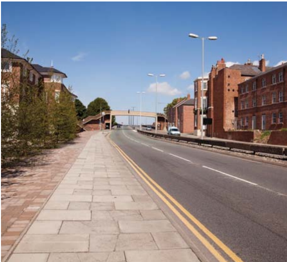
Highway lighting to the ring road
