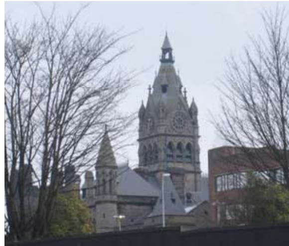
The Town Hall Tower is an important landmark with attractive features.
