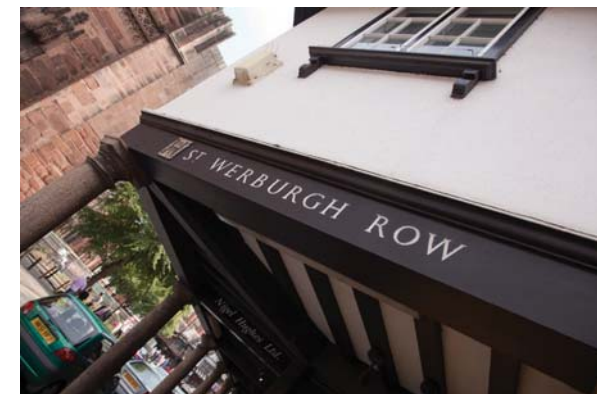
Example of street name painted onto buildings. These details should be retained and protected.
