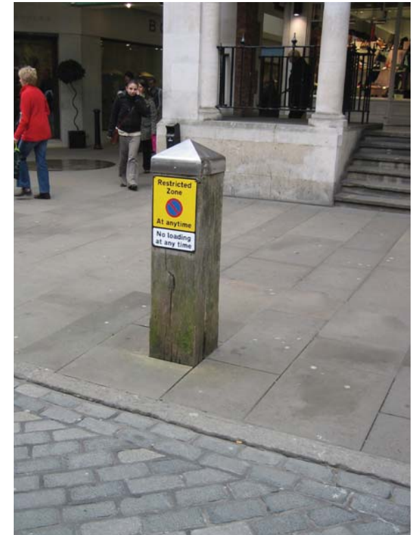
Example of signage mounted to bollard on street subject to traffic regulation order with a setted carriageway.
