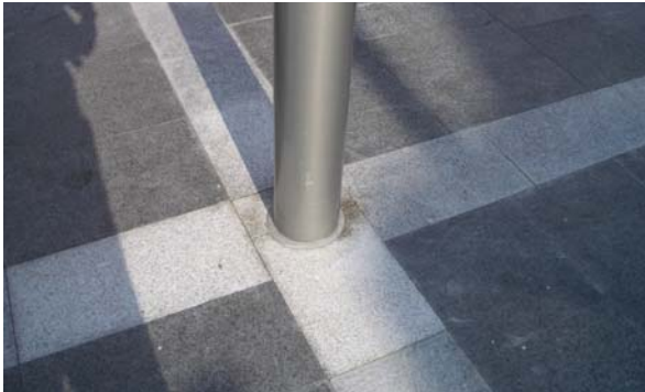
Good example of post positioned to neatly sit within paving layout, Berkley Square, Liverpool.
