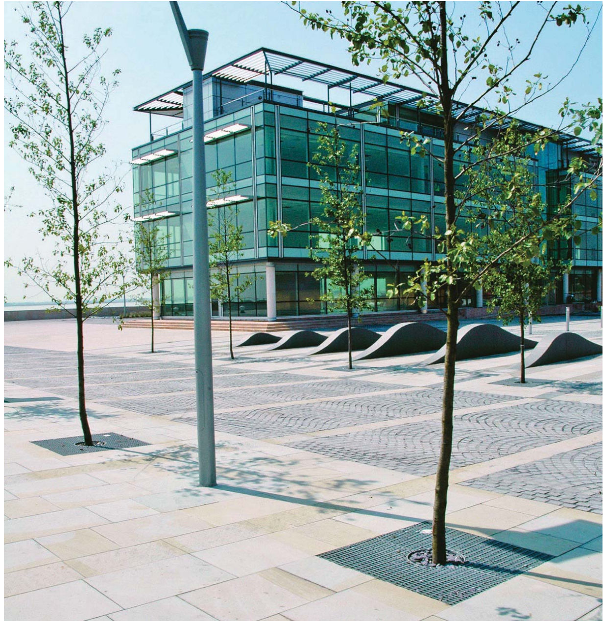
Example of well planned paving layout in Hull - paving units match and align with tree grilles.
