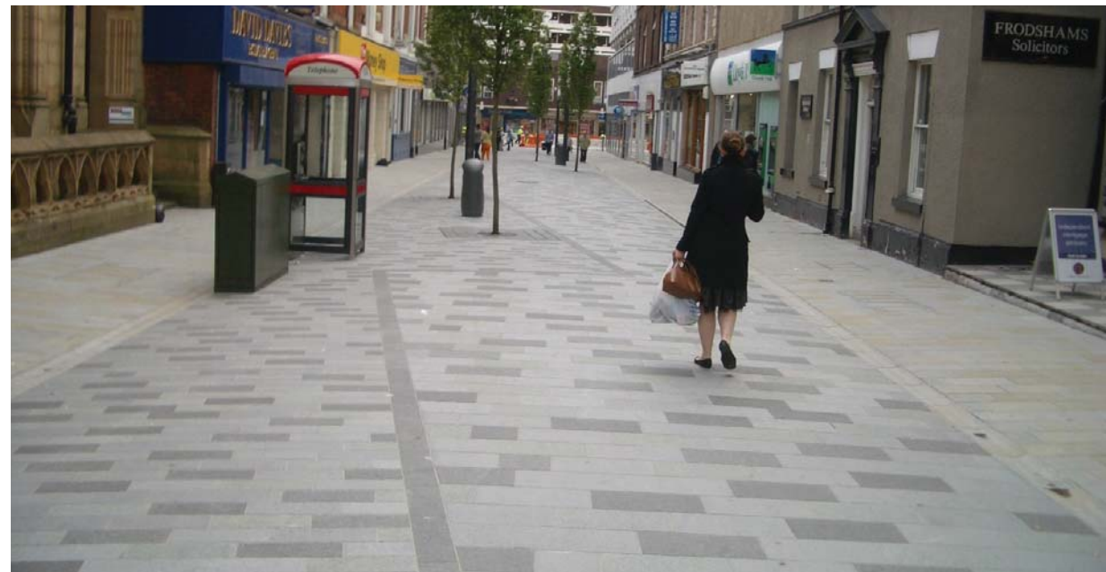
Paving during construction and following completion using rigid concrete construction, St Helens
