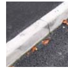
Standard Concrete Kerbs
