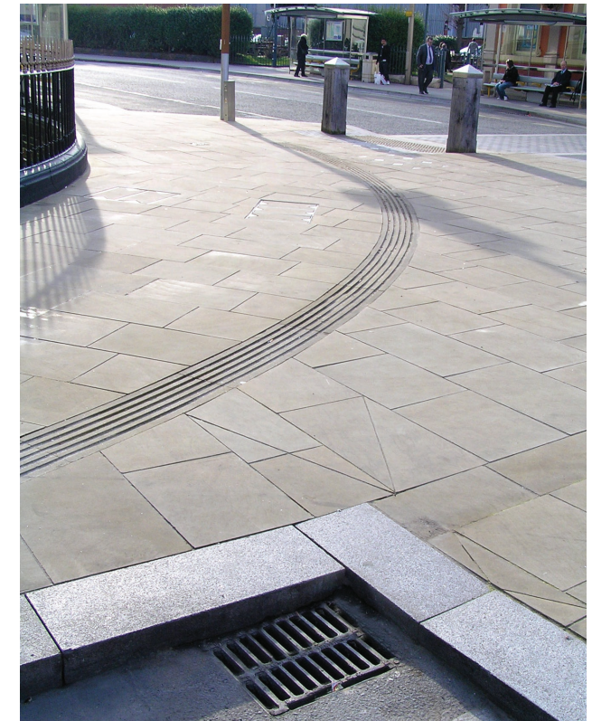
slotted drainage channel, outside station in Chester
