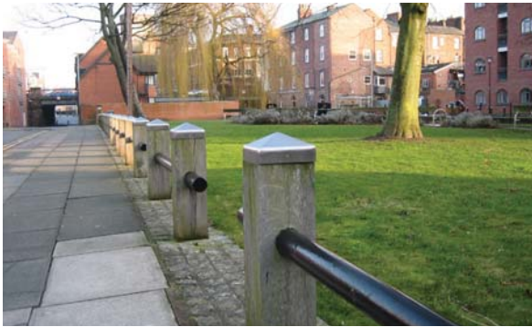
Timber post (with stainless steel cap) with powder coated steel (black) or stainless steel rail
