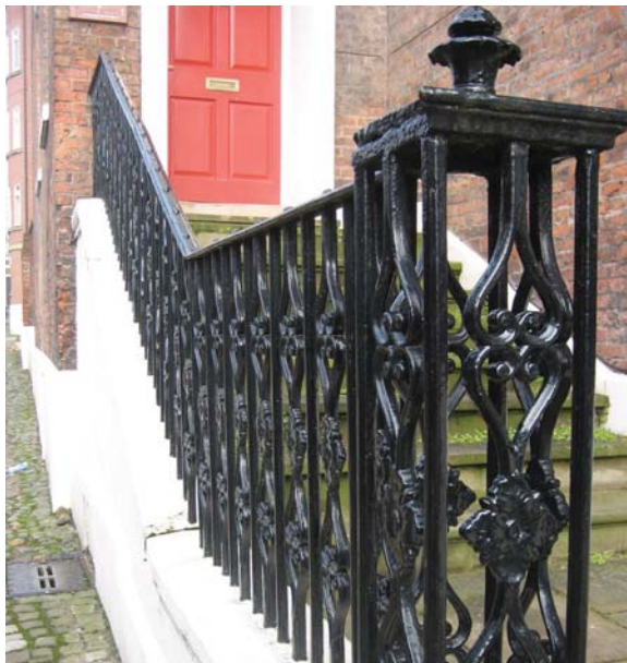
Examples of existing railings found in Chester City Centre
