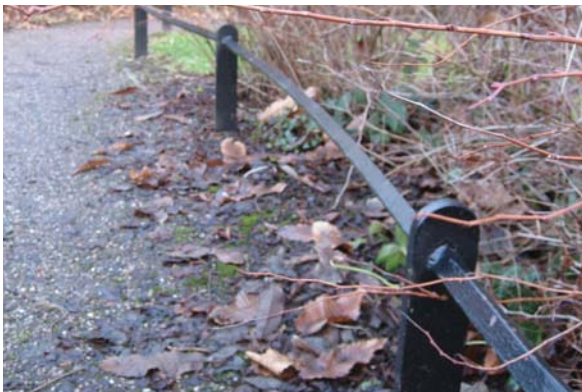
Powder coated galvanized steel post and rail (in black)
