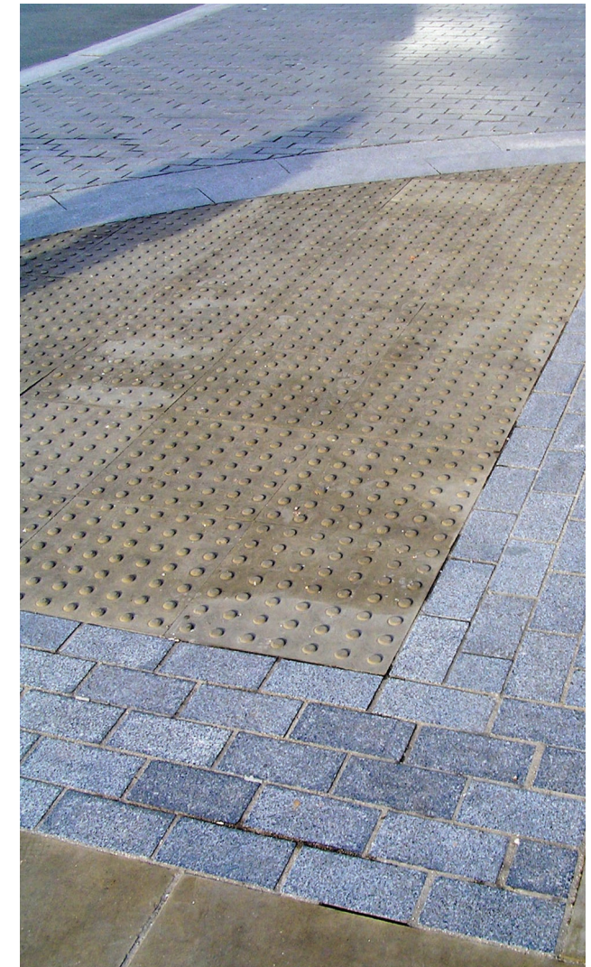
Existing natural stone tactile paving in Chester
