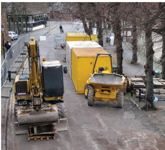
Public realm resurfacing at The Groves
