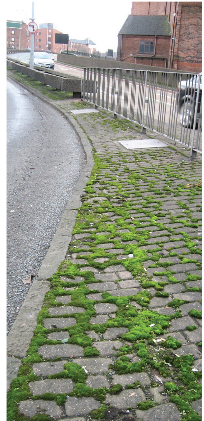
Weed Growth Between Setts on St Oswalds Way
