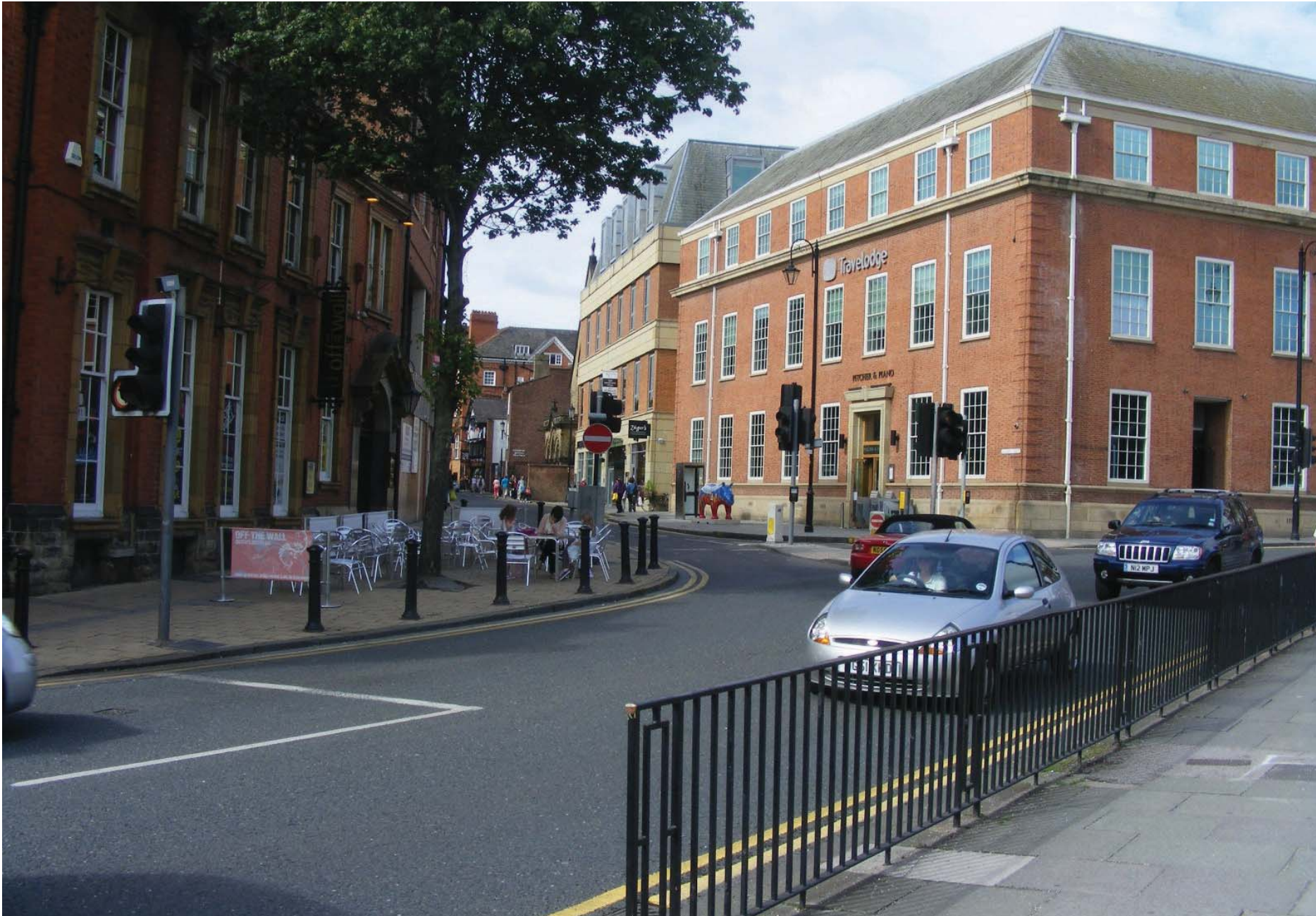
St John Street Existing (as viewed from Little St John Street)
