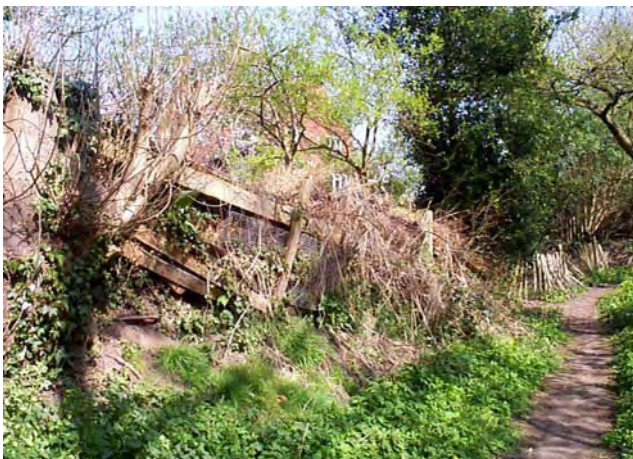
Compost heap pressure on fence near to Synagogue Well
