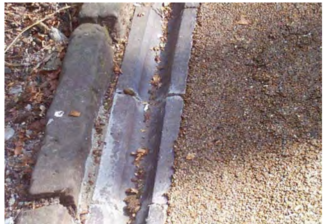
Drainage channel along path sides
