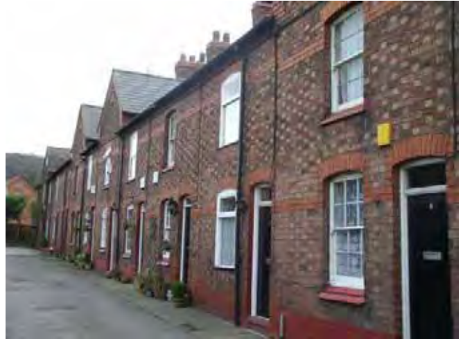
Moreton Terrace featuring pale-headed Flemish bond brickwork
