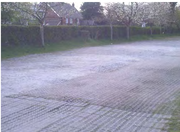
Failed reinforced grass car parking area
