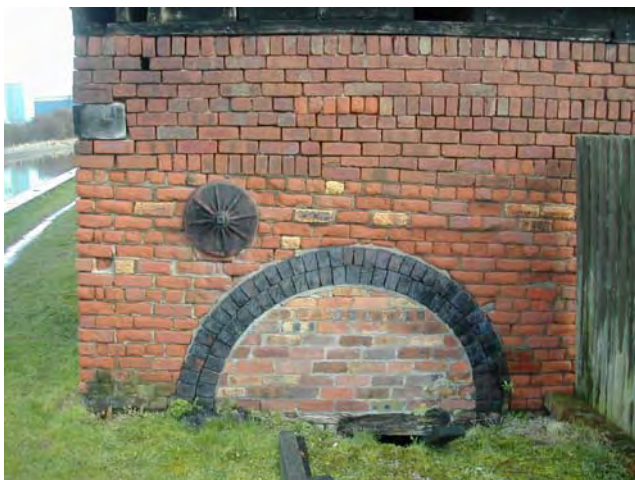
Ribbed cast iron structural tie plate
