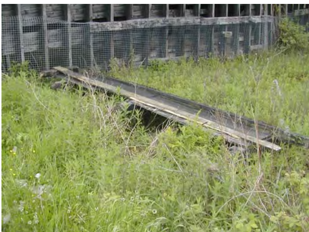
Damaged stop-plank housing
