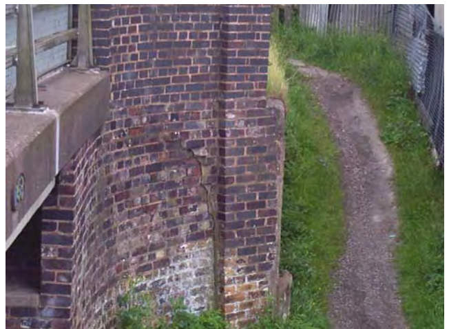
Stress crack in bridge abutment
