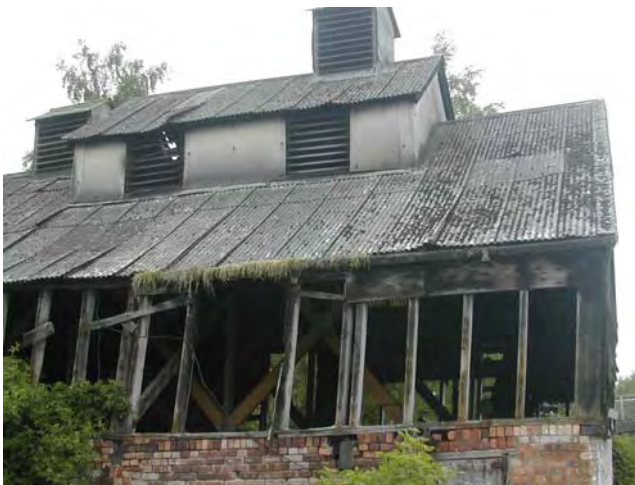
Roof hatches with ventilation louvers
