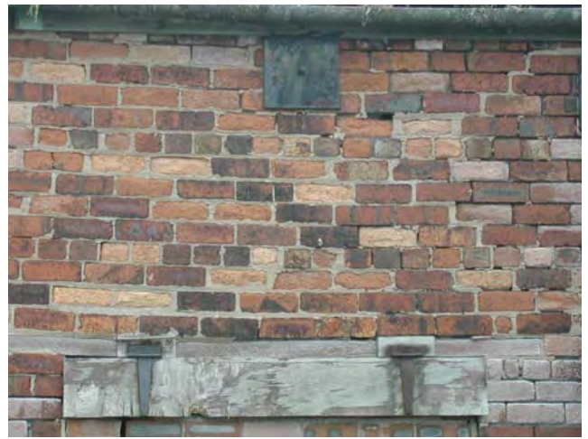
Timber flap with metal hinges and square wall tie plate
