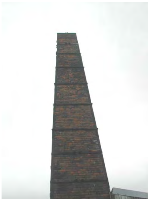
Tall Pump House chimney with iron strapping
