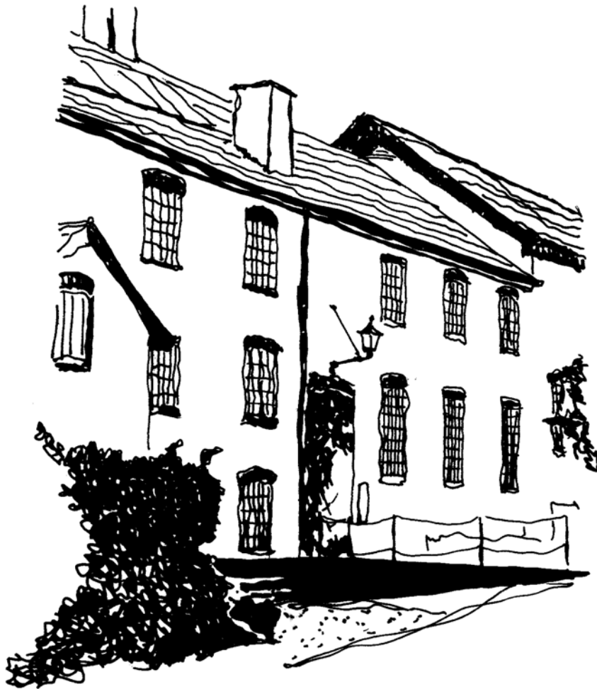
Former Canal Workshops
